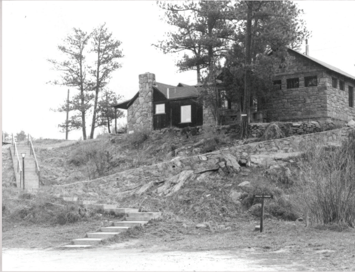
Original stone library and attached cabin
